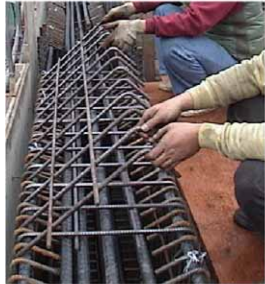
Figure 4 Construction of the Cap of Stirrup Cages
