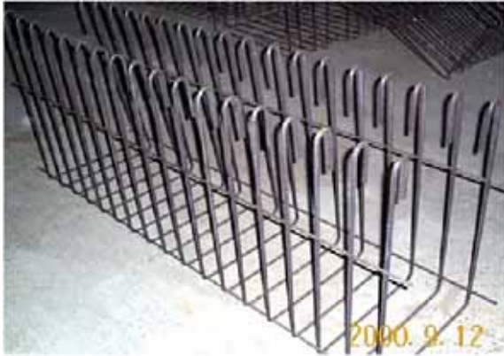
Figure 3 Stirrup Cage for Beams
